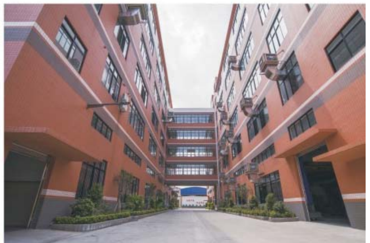
威浦局部厂区 Workshop building
